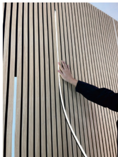
7. Fit the product into the panel groove.
