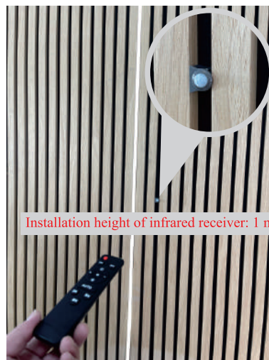
8. Mount the remote control receiver at a height of 100 cm above the floor
